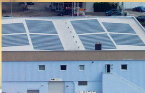
Centre Commercial, ▲ Wasserbillig, Luxembourg: 32,3 kW c
